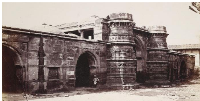
Fig. 1 Front view of Queen's Mosque showing fungal growth on the surface
